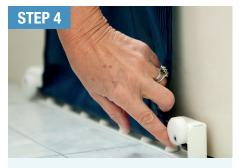
By rotating the discs the anchor bar can be located into the mounting bar itself. Turn the discs to ensure the anchor bar is positively locked in.
